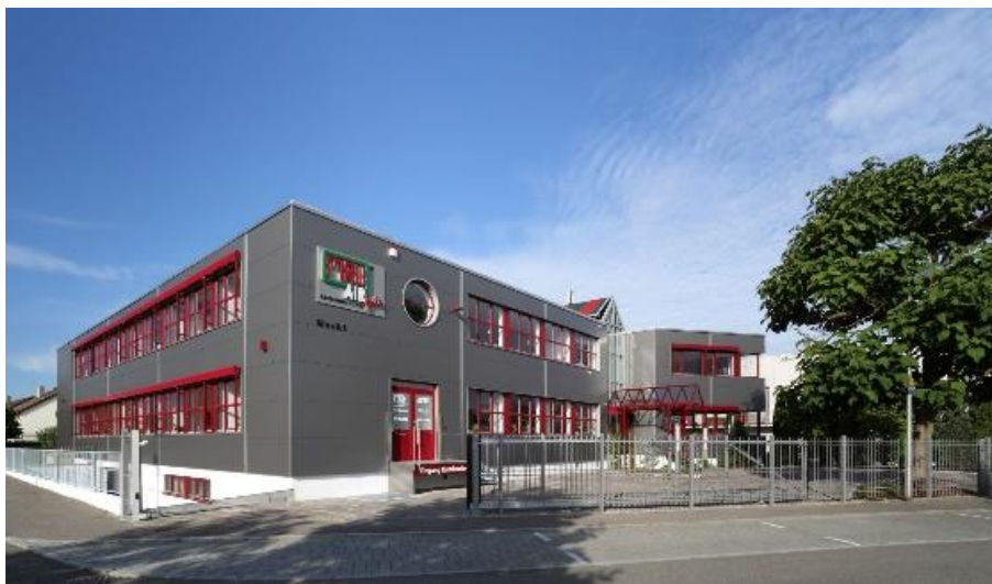
Building 1: Sales, Service, R&D
