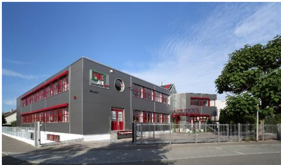
Building 1: Sales, Service, R&D
